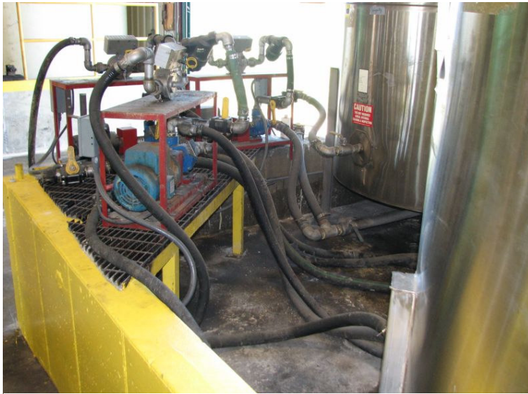
Figure 2. Example of Appurtenances Being Protected
